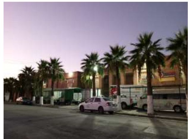
Figure 2 Torreón food bank facilities
